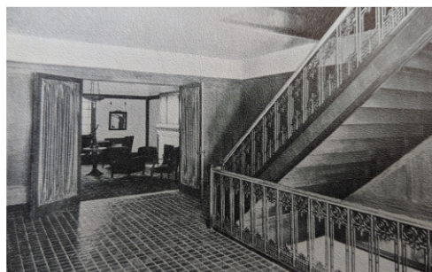
Stairway (Lodge Room Floor)
